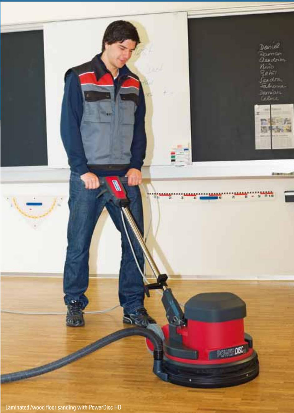
Laminated/wood floor sanding with PowerDisc HD
